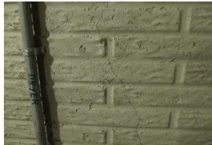
minor crack in wall at 2109 Chapel - stabilize grade and monitor for continued movement
