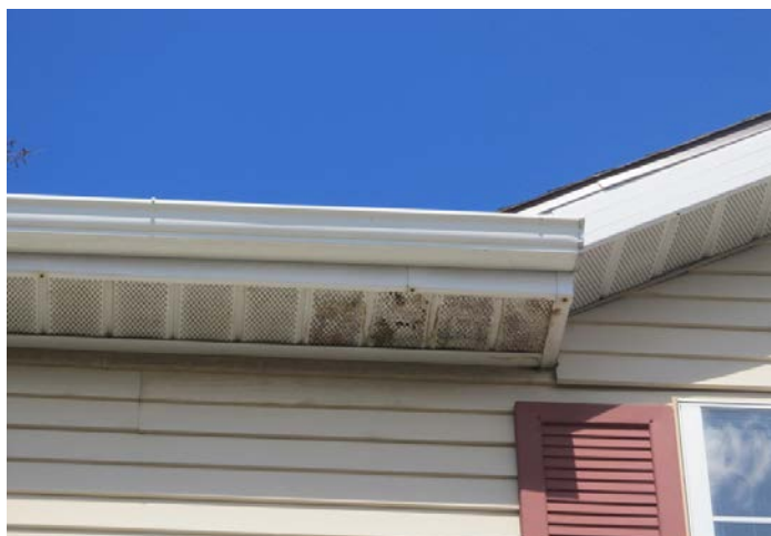
soffit deterioration at 2127 Chapel
