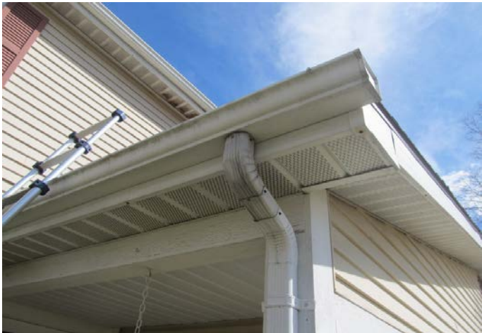
aluminum gutter and downspout
