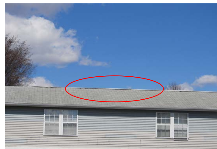
example of ridge vents improperly continuous between units
