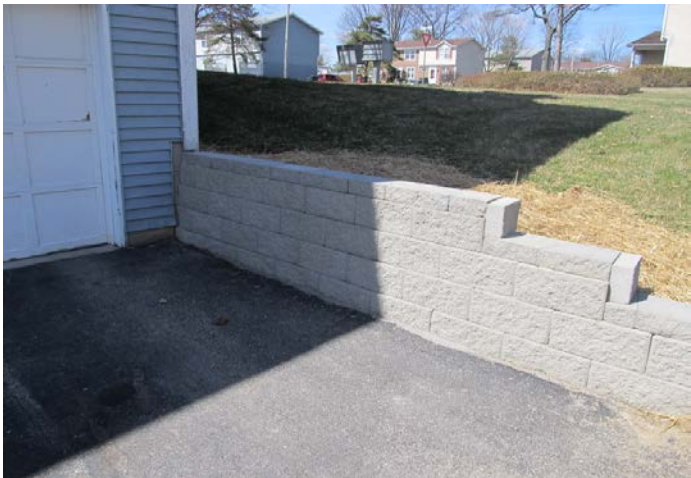
recently replaced masonry retaining wall
