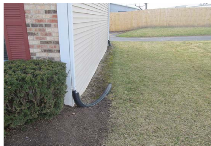
lack of grading away from building at 2161-2167 Chapel
