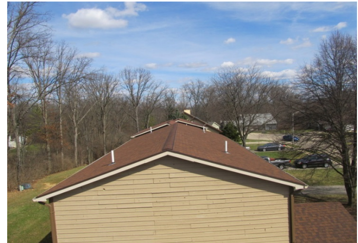
roof with asphalt shingles
