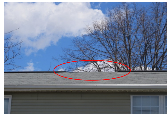
example of ridge vents properly not continuous between units
