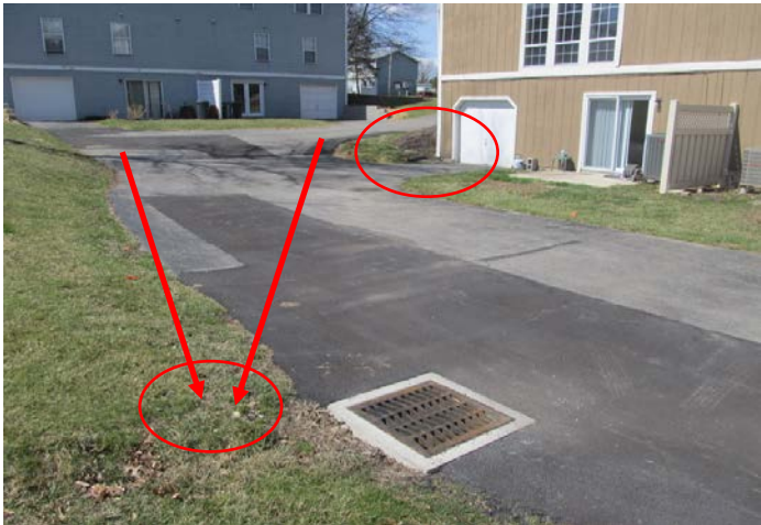
catch basin at 410-412 White Ash is inadequate for drainage of pavement resulting in flooding of the adjacent garage - regrade pavement and install French drains
