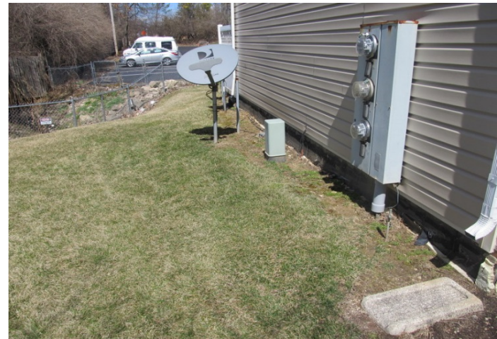
grade settlement and erosion towards stream at 2109 Chapel
