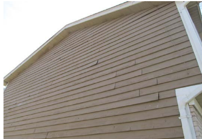
wood siding deterioration
