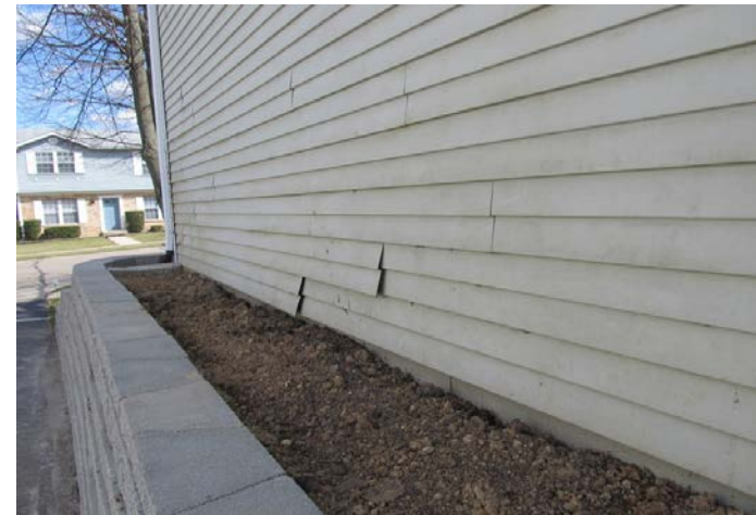
loose aluminum siding
