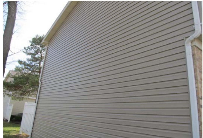
vinyl siding with Dutch lap profile
