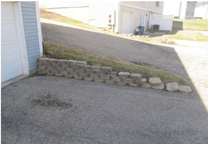
dated and failing retaining wall
