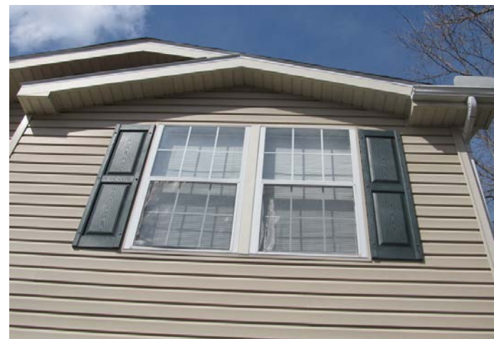
vinyl shutters with 6 fasteners per panel
