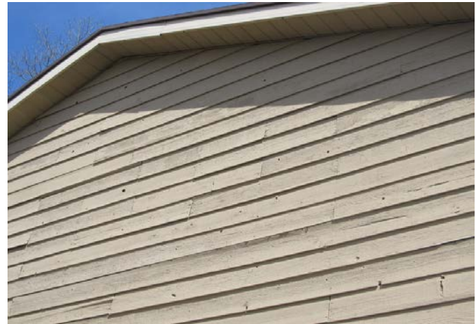
wood siding deterioration
