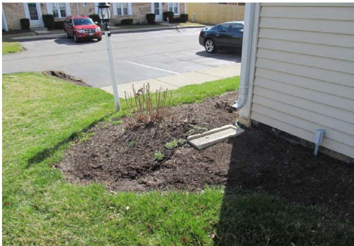
downspout too high off ground causing excessive splashing and erosion
