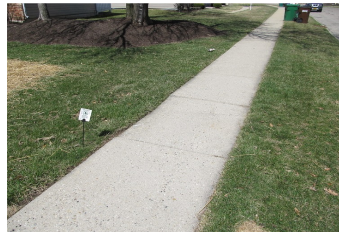
settled sidewalk section at 2105 Chapel
