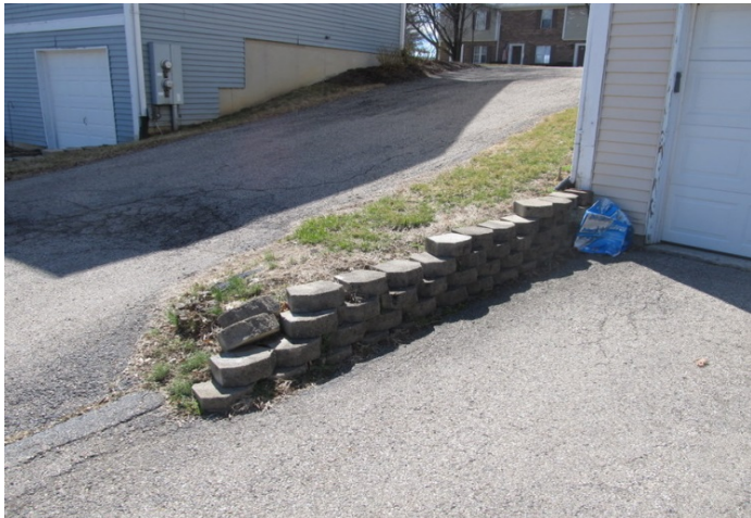
dated and failing retaining wall
