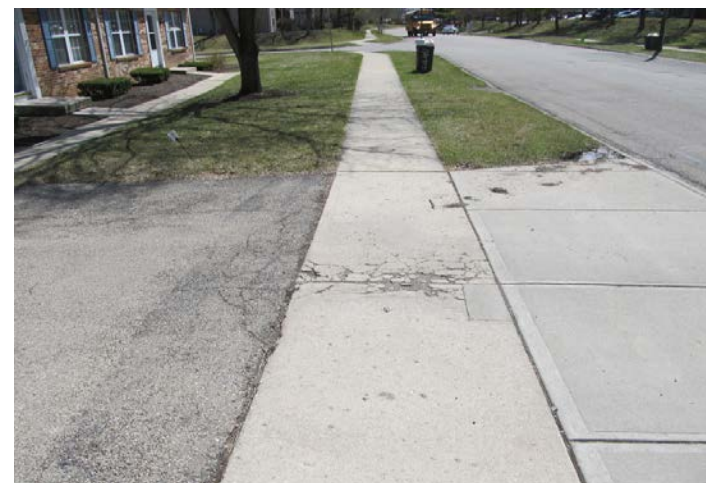
sidewalk deterioration at 2172 Chapel
