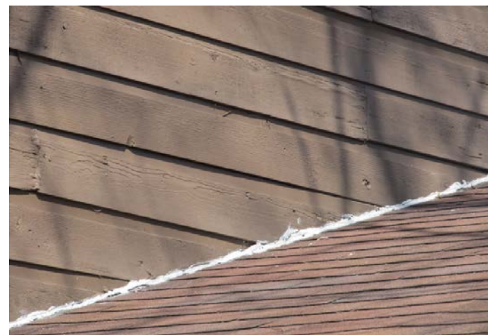
siding in contact with the roof (properly installed step flashing with the shingles and siding does not require caulk at this location)
