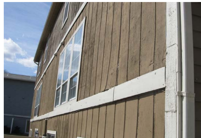
plywood siding deterioration
