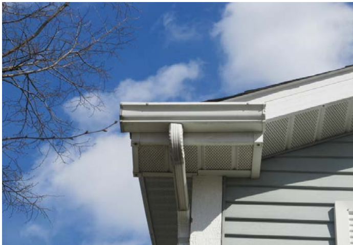
aluminum gutter and downspout
