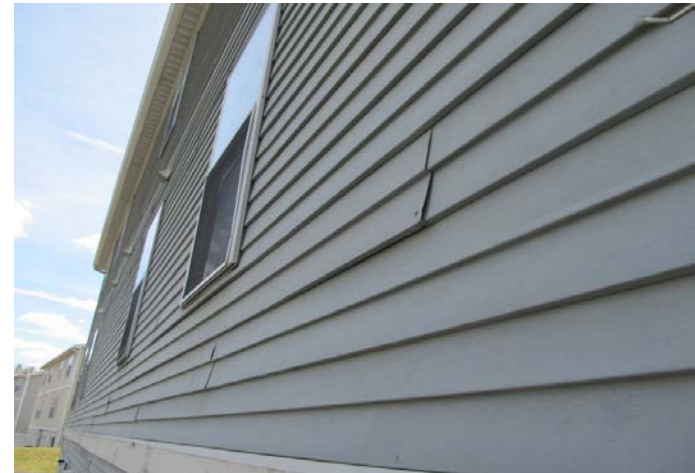
aluminum siding with double clapboard profile
