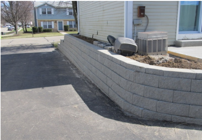
recently replaced masonry retaining wall
